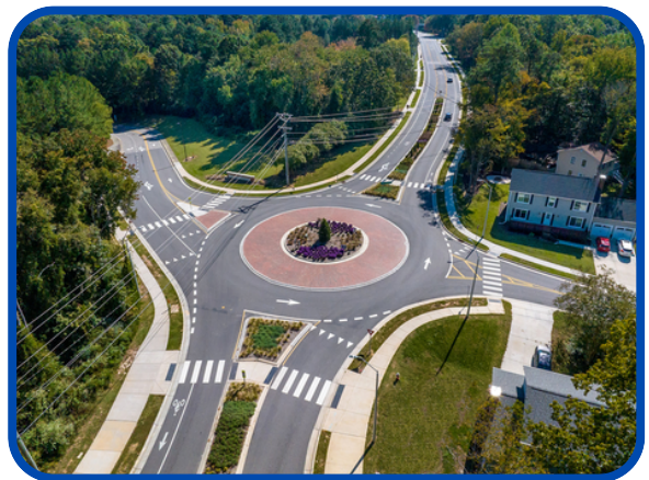
Town of Cary new roundabout.
