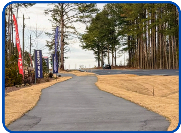
Newly constructed paved sidepath along Matthews Road
