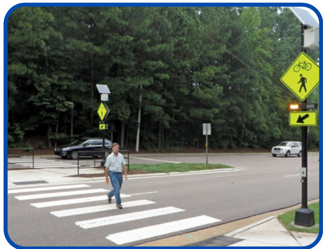
Example of a high-visibility crosswalk
