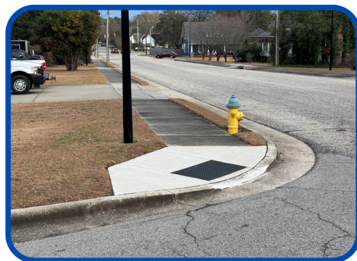
New curb ramp at an intersection.
