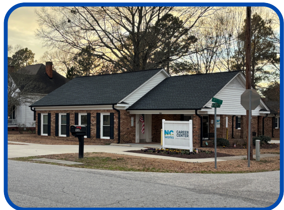
Adaptive reuse of a residential property near downtown Lillington.
