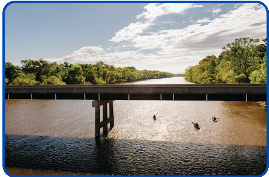
NC 401/421 Bridge over Cape Fear River.
