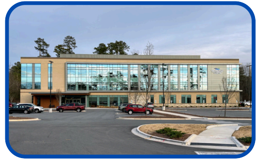
Recently built Cape Fear Valley Cancer Center
